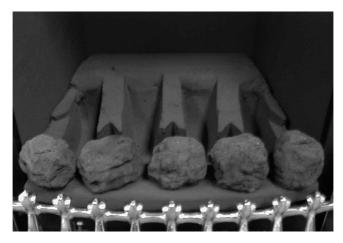
d) Select four of the large coals and arrange behind the front row of coals, ensuring that flame paths as indicated below are not interupted. (See fig. 13 below)
